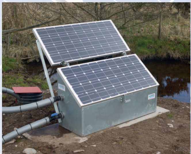
Figure 6: Packaged solar pump unit.
