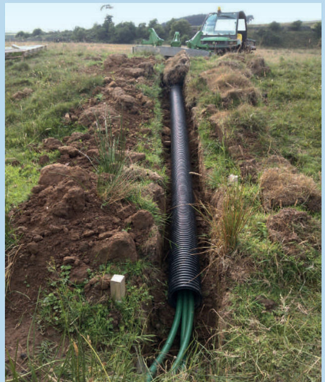
Figure 4: Installation of the underground transfer duct to protect suction hoses.
