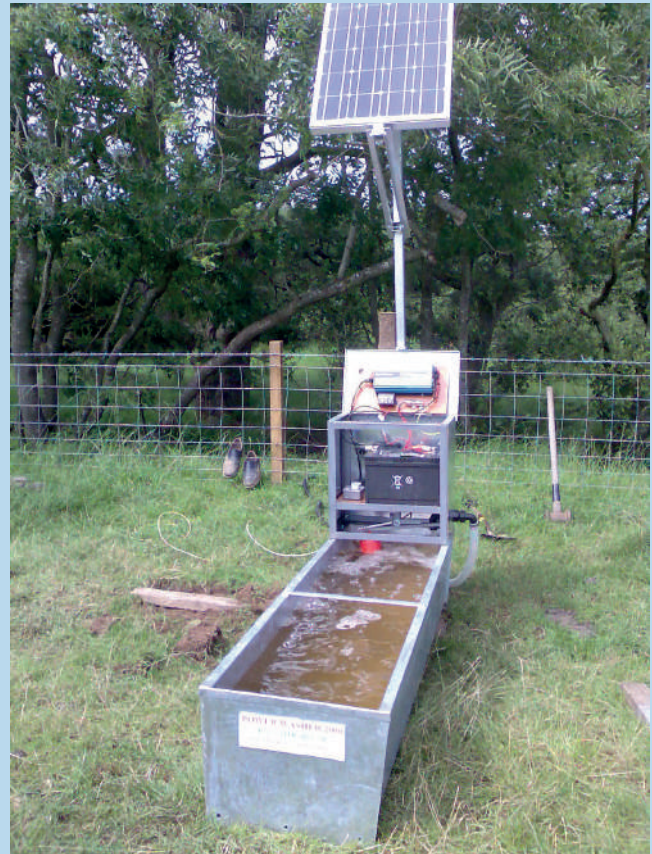
Figure 8: Solar system during installation. Covers removed showing battery compartment.
