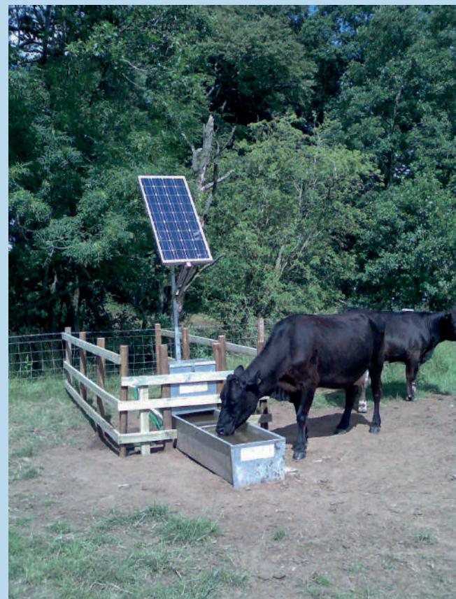
Figure 9: Livestock using trough. Fencing only part completed but prevents access to battery and panel.
