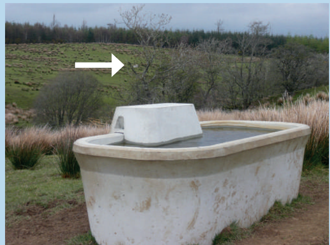
Figure 13: Water trough supplied by ram pump. Arrow indicates position of second trough.
