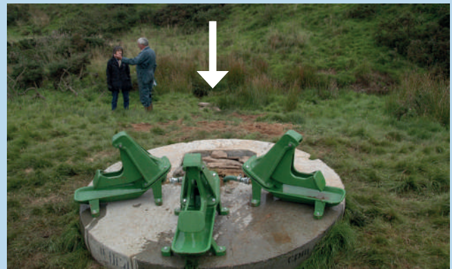
Figure 3: Pasture pump cluster looking towards watercourse. Arrow indicates position of abstraction point.
