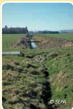
Field drainage systems
